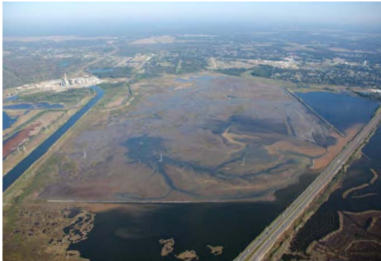
Figure 5: Aerial image of the beneficial uses site in November 2011, near the completion of dredge placement. View is looking north from Highway 73; containment terraces are visible along the edge of the site.
