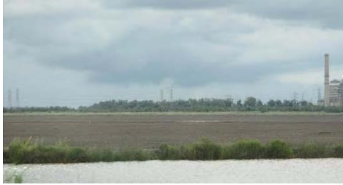
Figure 7: View of dredge material in the beneficial uses site in June 2012, showing the unvegetated terrain.
